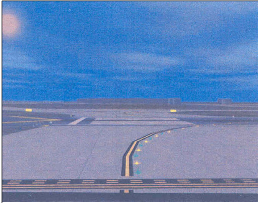
FIG 2-1-12 Taxiway Lead-On Light Configuration
