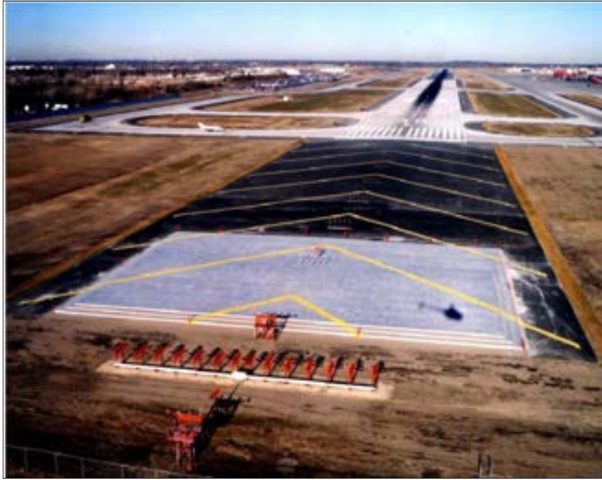
FIG 2-3-42 Engineered Materials Arresting System (EMAS)
